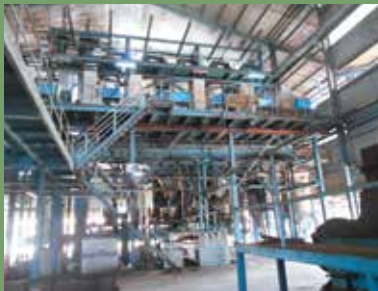
Oil Mill at PT Rebinmas Jaya, Pulau Belitung
